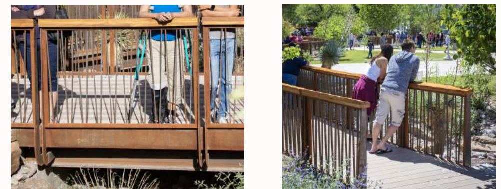
Railing: Corten Steel and Wood
