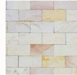
Commercial Hardscape use of split stone paving
