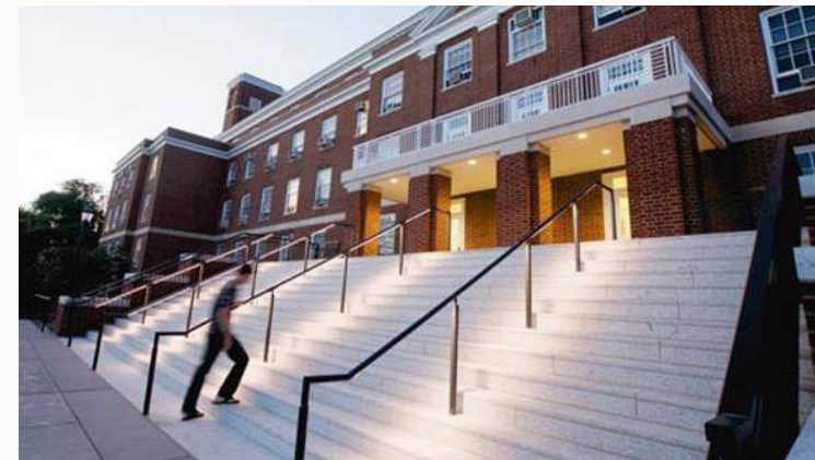
Handrail integrated lighting help define the steps and provides for a unobstructed path.
