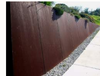
Corten Steel Retaining walls and planting zones
