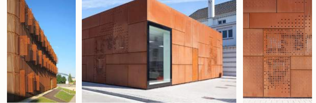
Bold, geometric shapes for architectural volume: consider corten steel as solid, perforated, with louvers.
