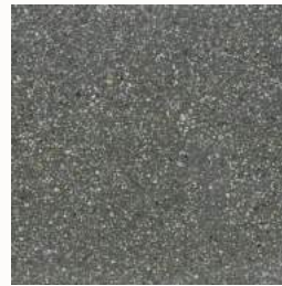
Cast In Place Concrete, or pavers Finish No. 5 Base Light Gray, Ecocast 3 Light Grey Integral Color (Trademark) Acacia Square Hardscape
